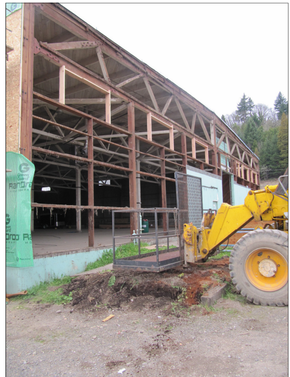
Construction crews bringing our new warehouse back to life.
